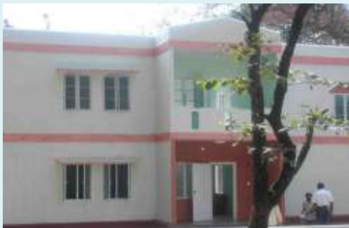
Two storey Construction of First Rapid wall Building in India in Mumbai in 32 days by RCF (structural design by IIT Madras)
