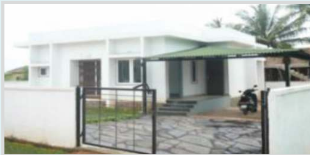
Rapid wall Residential building at Mumbai
