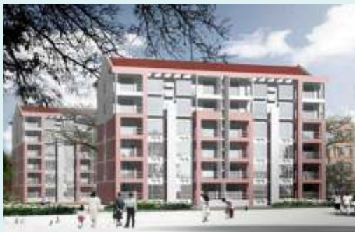
Seven storey Apartment Gypcrete building in Tianjin, China.
