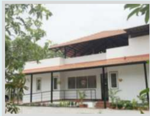
Rapid wall Courtyard Home in Vellore
