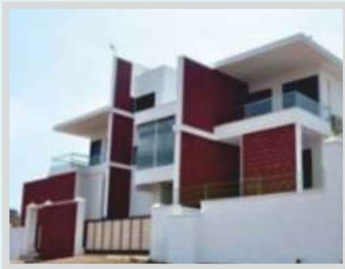
Rapid wall 2 storeyed Residential building at Manipal
