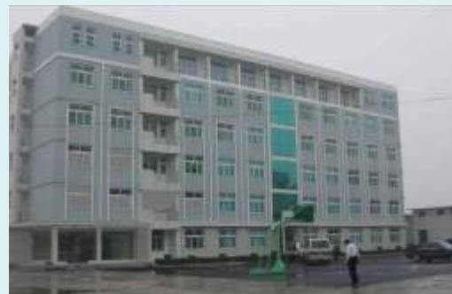
Six storeyed Guest House building in an industrial park in Jinan city, Shandong Province, China.
